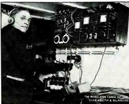
Ships had used 1000 kHz for a long time prior to the creation of the broadcast band. It took a few years to work out all of the details, but the broadcasters won out and the many coastal stations and vessels were banished. This 1925 photo shows the radio shack aboard the 40-ft. motor lifeboat "Elizabeth & Blanche."
